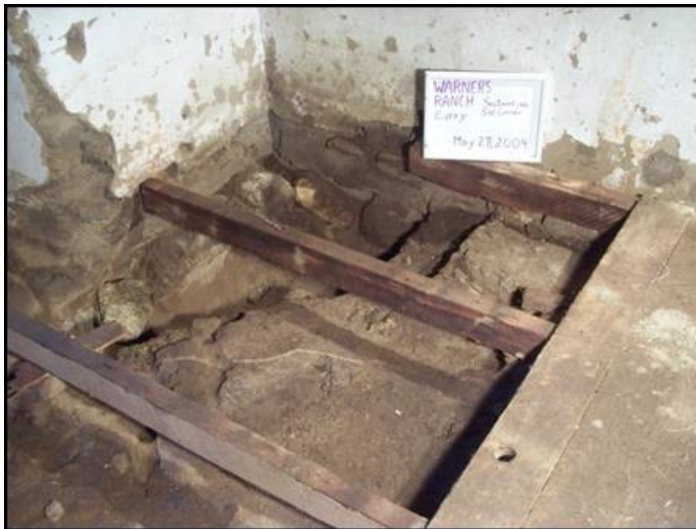
Figure 10.42. Overview of the excavation unit in the southwest corner of Excavation Block Section 6. Note the single course of large irregular shaped granite field stones in the foundation. Courtesy Stephen R. Van Wormer and Susan D. Walter.
