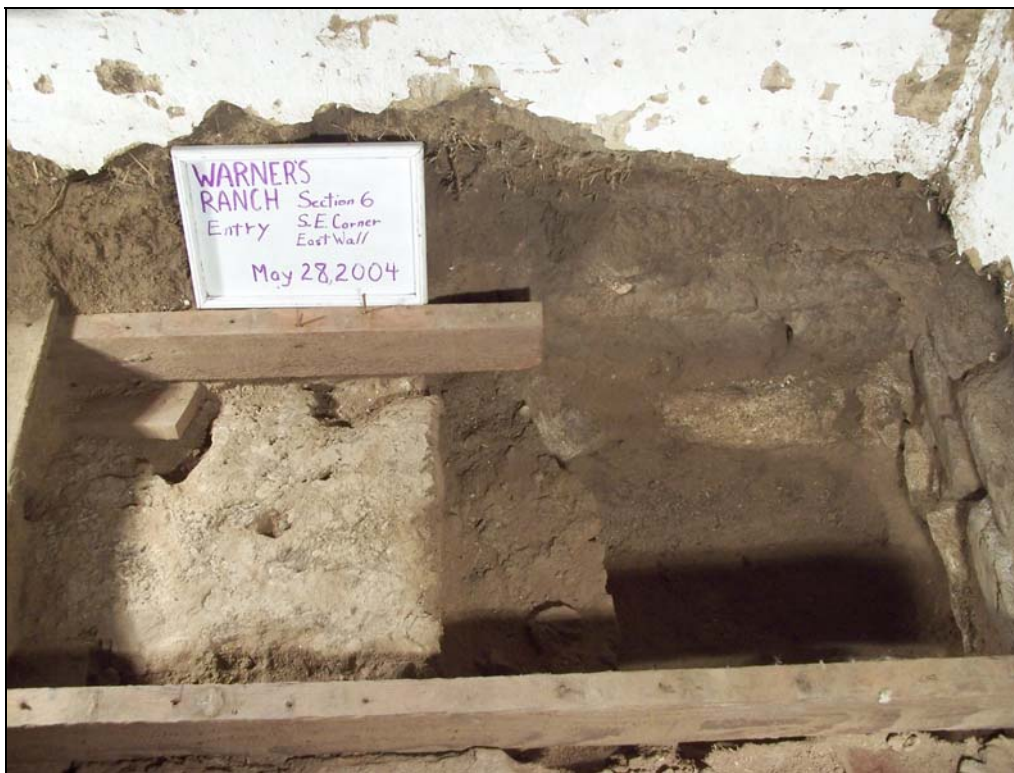
Figure 10.37. Entry Room Excavation Block Section 6 following excavation of the northeast corner, looking east. A portion of the far sleeper has been cut off to allow excavation access. Note (A) the present wooden floor board, (B) sleepers, (C) upper earthen floor, (D) lower earthen floor, (E) adobe blocks at the base of the wall, and (F) a single course of field stones underlying the wall.
