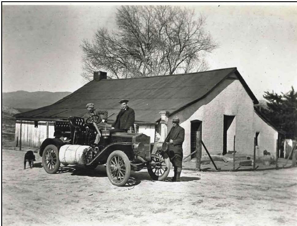
Figure 10.14. Photograph of the ranch house circa 1910. Note the board and batten siding along the south side and the masonry steps and facing along the base of the east wall. Courtesy Stephen R. Van Wormer and Susan D. Walter.
