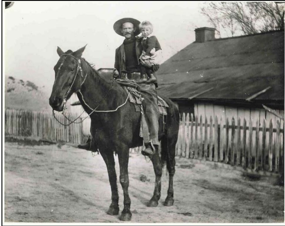
Figure 10.13. Sam Taylor and son in front of the ranch house in 1904. Note the board and batten siding along the south wall. Courtesy San Diego Historical Society.
