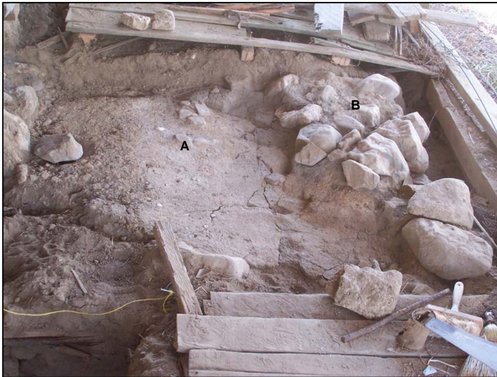
Figure 10.24. An area of the original porch cleared of debris. Note the hard packed earthen surface that appears to have been laid as a mud slurry (A) and the shallow cobble footing at along the north edge (B). Courtesy Stephen R. Van Wormer and Susan D. Walter.
