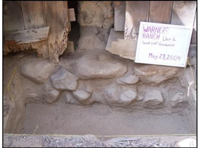
Figure 10.4. Cobble foundation and the end of the western interior dividing wall in Unit 2. Courtesy Stephen R. Van Wormer and Susan D. Walter.
