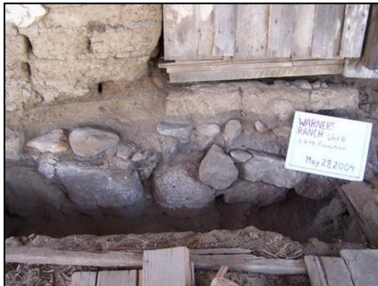
Figure 10.20. The stone foundation and the bottom course of the original adobe wall in Unit 6 underlying the northern wall wooden infill. Courtesy Stephen R. Van Wormer and Susan D. Walter.
