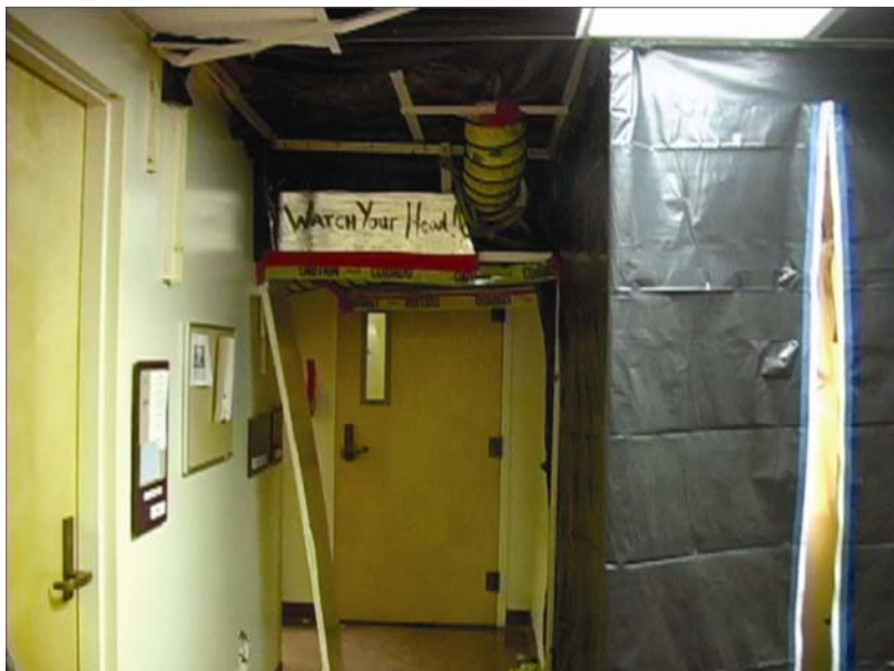
Figure 5.12. The finished ventilation system. Courtesy of Seth Mallios and Donna Byczkiewicz.
