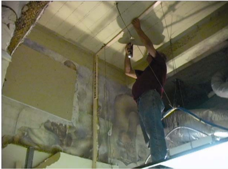
Figure 5.11. Zakheim constructs a wooden frame around the mural area. Courtesy of Seth Mallios and Donna Byczkiewicz.
