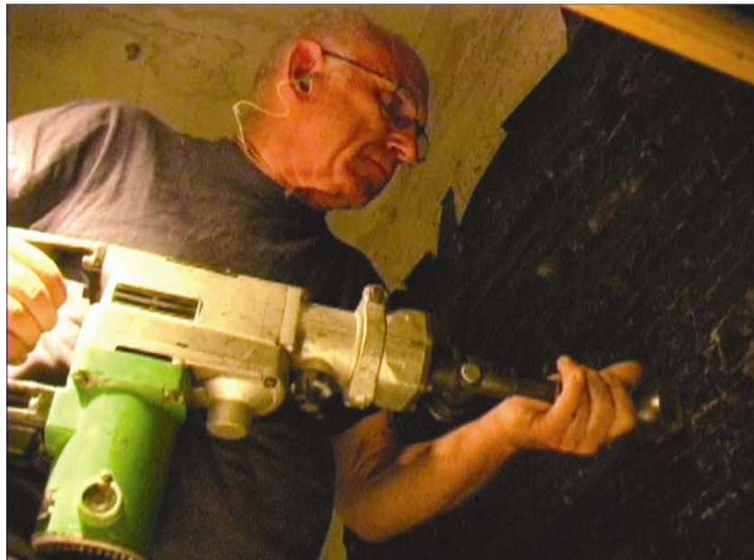
Figure 5.18. Zakheim uses an air hammer to send vibrations through the mural and into the concrete wall. Courtesy of Seth Mallios and Donna Byczkiewicz.
