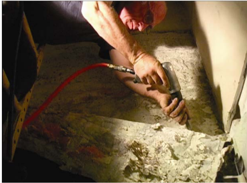
Figure 5.19. A chisel is used to peel the back of the mural down the wall after the air hammers have started the fissuring process. Courtesy of Seth Mallios and Donna Byczkiewicz.
