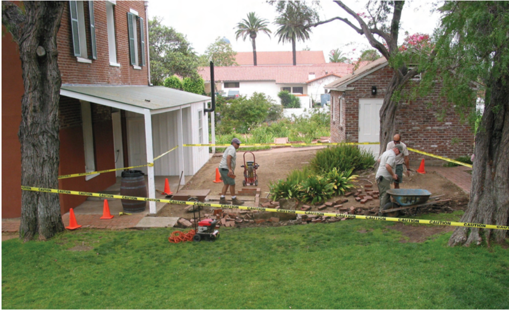
Figure 7.7 County workers remove the brick path, concrete pads, and plants that would interfere with the ground-penetrating radar. Courtesy Seth Mallios, David Caterino, and the South Coastal Information Center.
